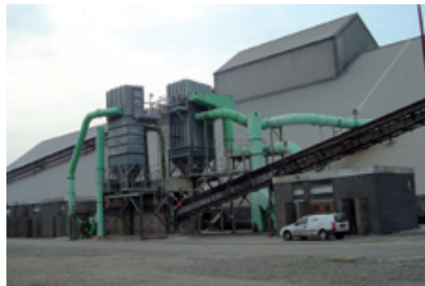
Bag filters found on Electrolytic reduction and smelting processes utilise networked DT990 systems
