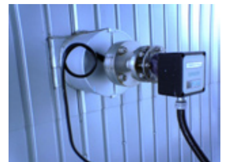
Dynamic Opacity monitor approved to TÜV / MCERTS fitted to an electro-filter stack
