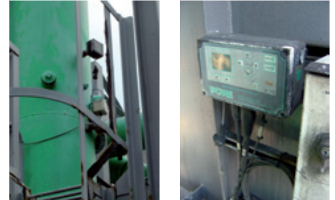
Anode baking plant monitored by a TUV approved Electrodynamic system
