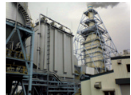
Dynamic Opacity monitor used to monitor electro-filter after calciner
